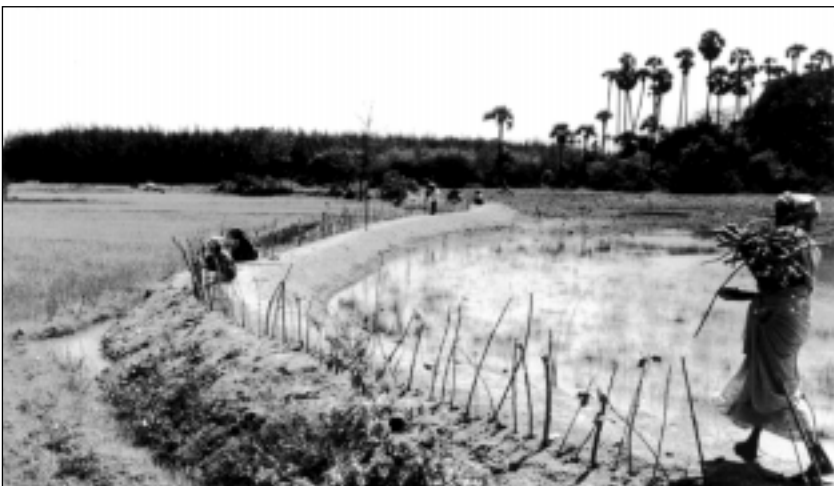
A recently constructed water catchment check-dam near Thuruwai village
