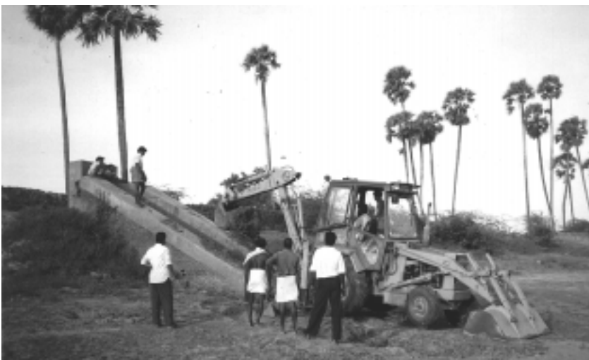
Working on renovation of a sluice
