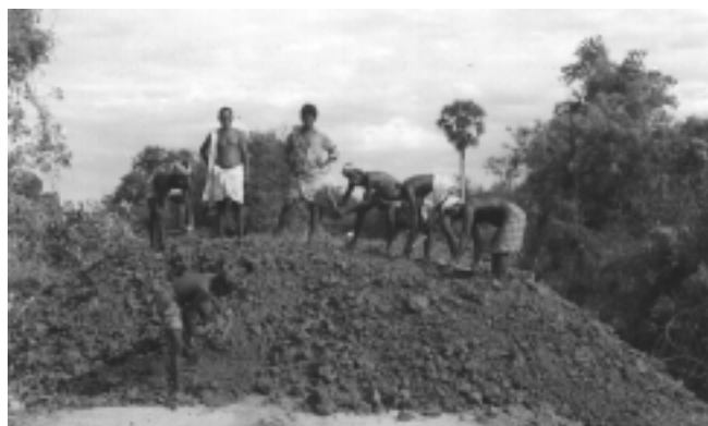
Raising a water catchment tank wall by over a metre
