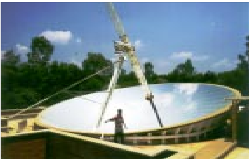
15 metre diameter solar collector on roof of Solar Kitchen
