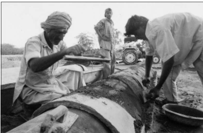
Fabricating Auroville-designed roof channels in Gujarat
