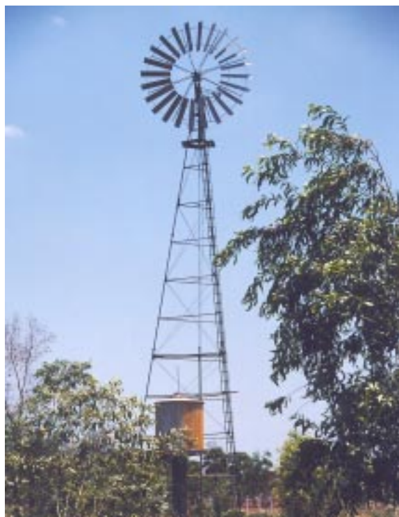
An AV55 in Auroville's Botanical Garden, one of many used to pump up water in the township area
